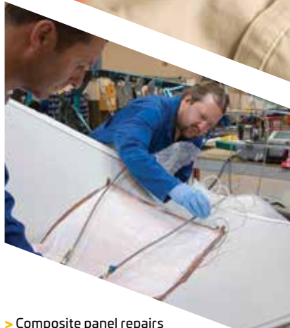
> Composite panel repairs
